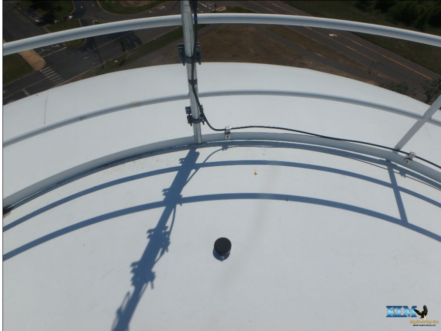
Photo No. 45 Condition of the roof and handrail
