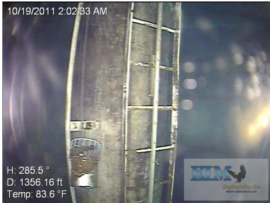
Photo No. 11 Drywell tube, ladder, and mixer
