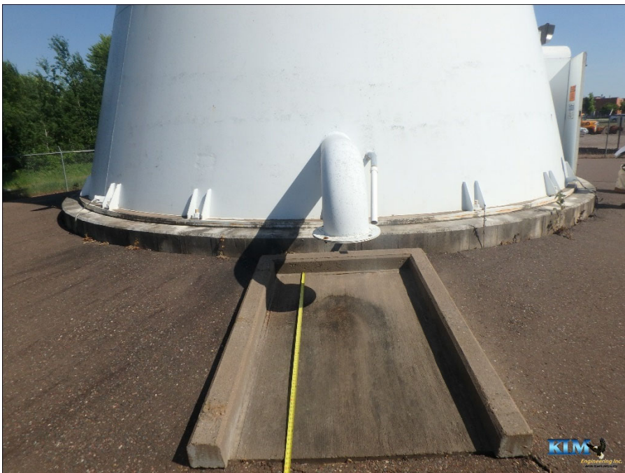
Photo No. 58 Base cone, overflow pipe outlet, and splash pad
