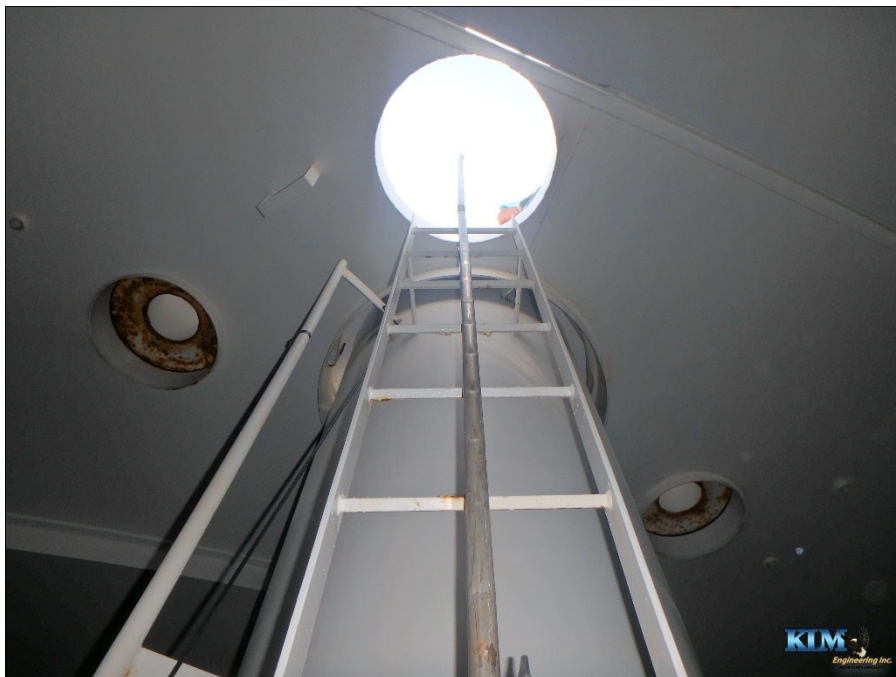
Photo No. 2 Upper interior wet ladder, drywell tube, and roof
