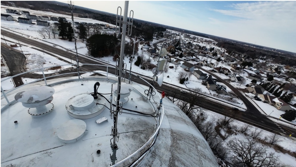
Photo No. 47 View of roof Taken in 2026
