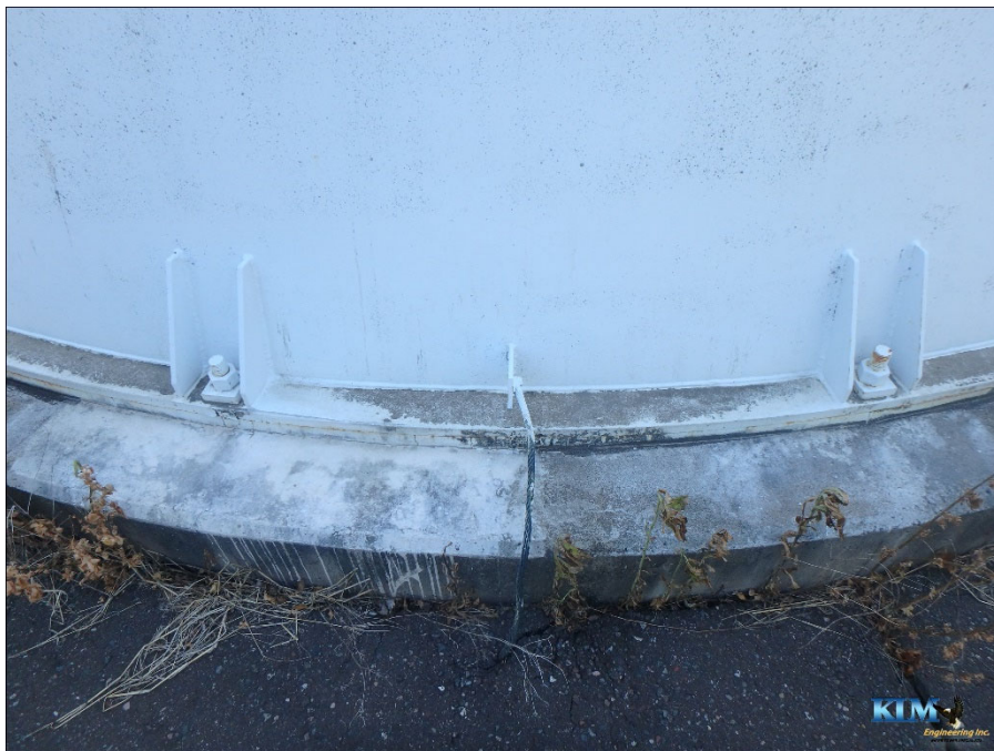
Photo No. 56 Tower base plate and foundation
