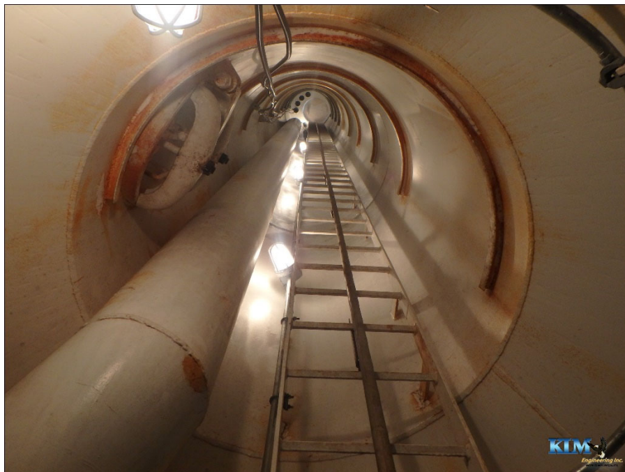
Photo No. 24 View at bottom of drywell tube looking up Manway visible
