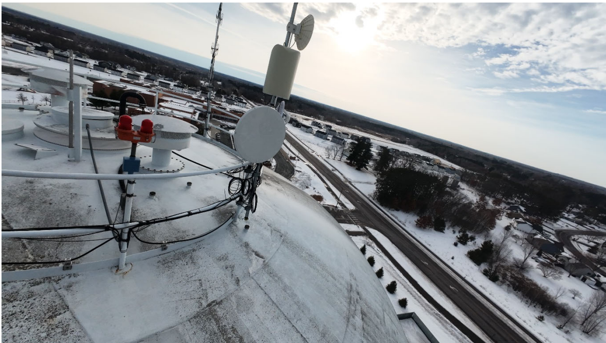
Photo No. 48 View of roof Taken in 2026
