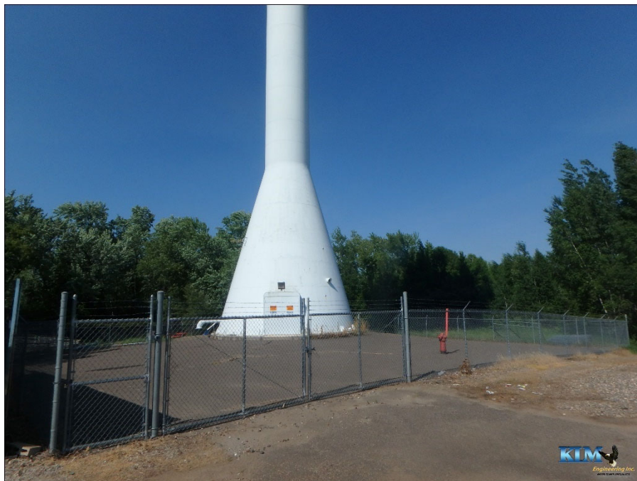
Photo No. 60 Site conditions
