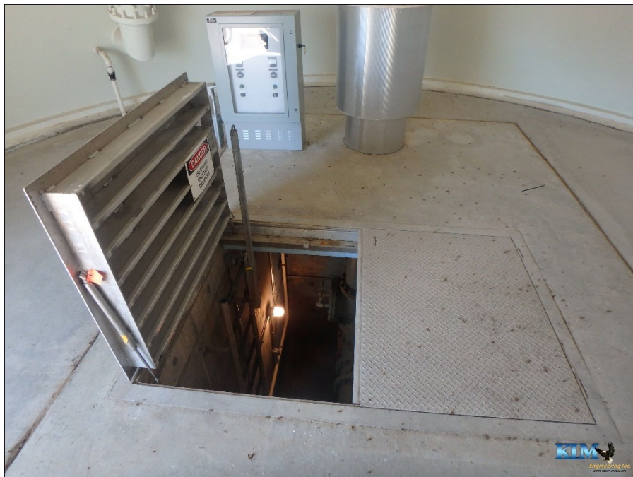
Photo No. 40 Valve pit access
