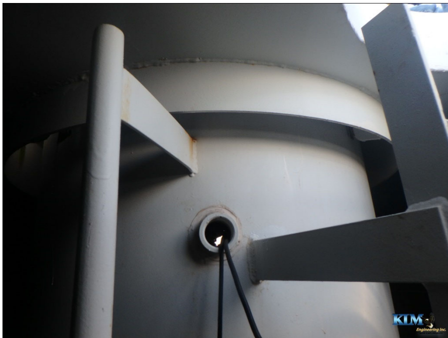
Photo No. 4 Top of the drywell tube with mixer cable penetration
