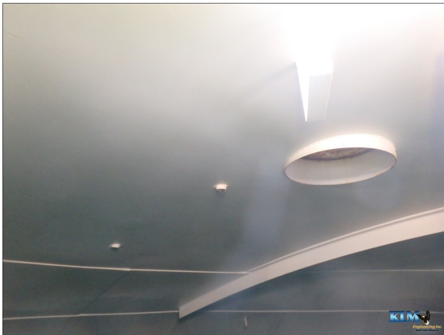
Photo No. 6 Condition of the roof
