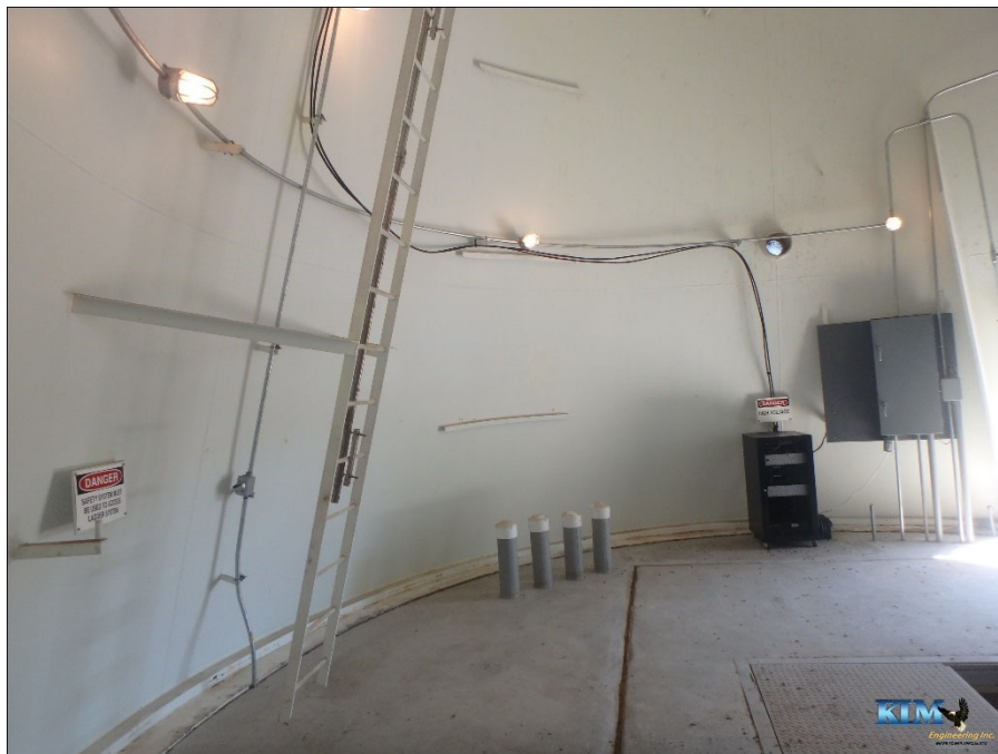
Photo No. 36 Condition of the base cone
