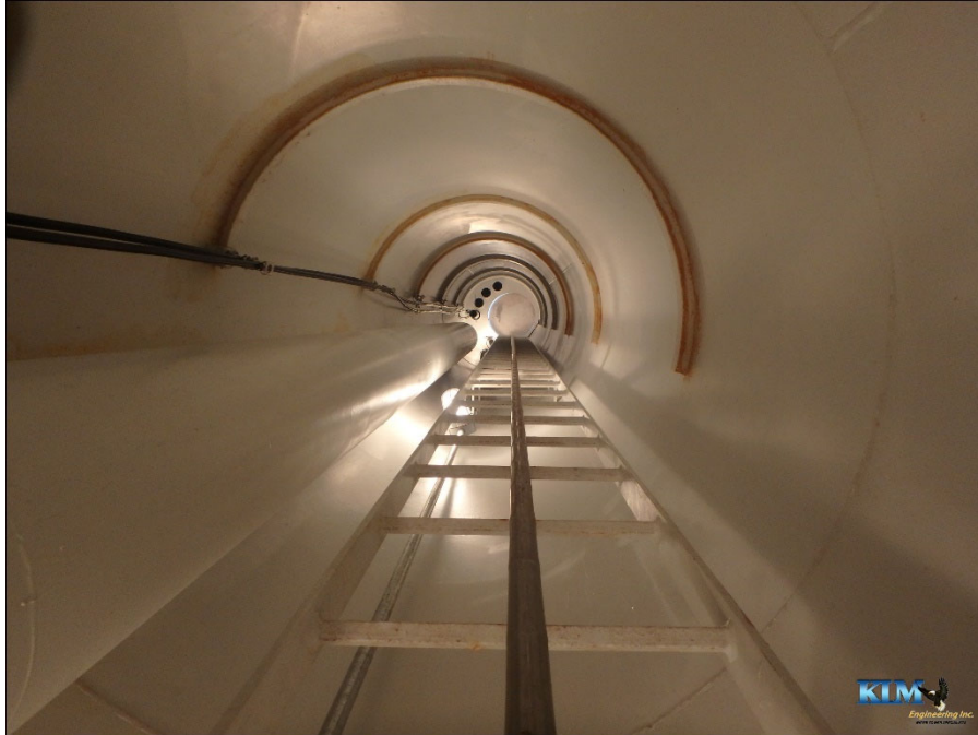
Photo No. 23 View inside the drywell tube looking up
