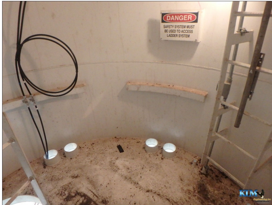
Photo No. 33 Condition of the pedestal and bottom landing
