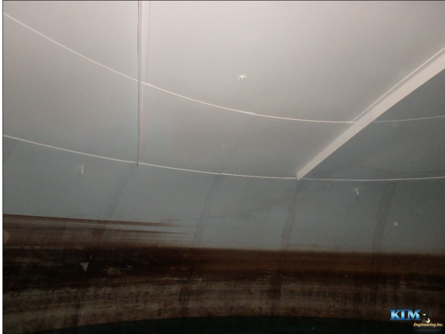
Photo No. 7 Condition of the roof
