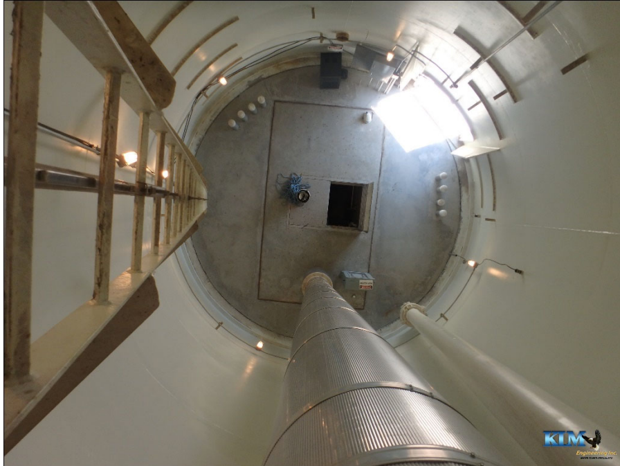
Photo No. 35 View of tower base
