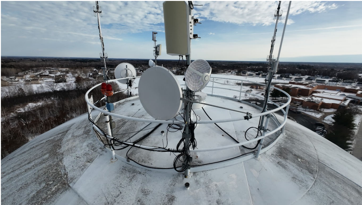
Photo No. 49 View of roof Taken in 2026
