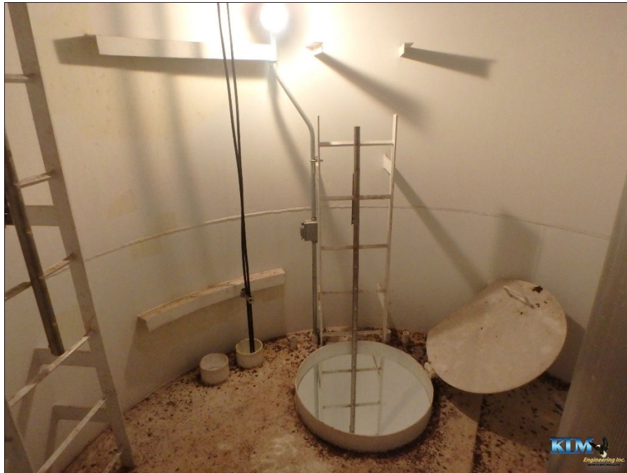
Photo No. 31 Condition of the pedestal and intermediate landing
