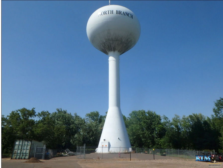
Photo No. 1 Overall view of the tower
