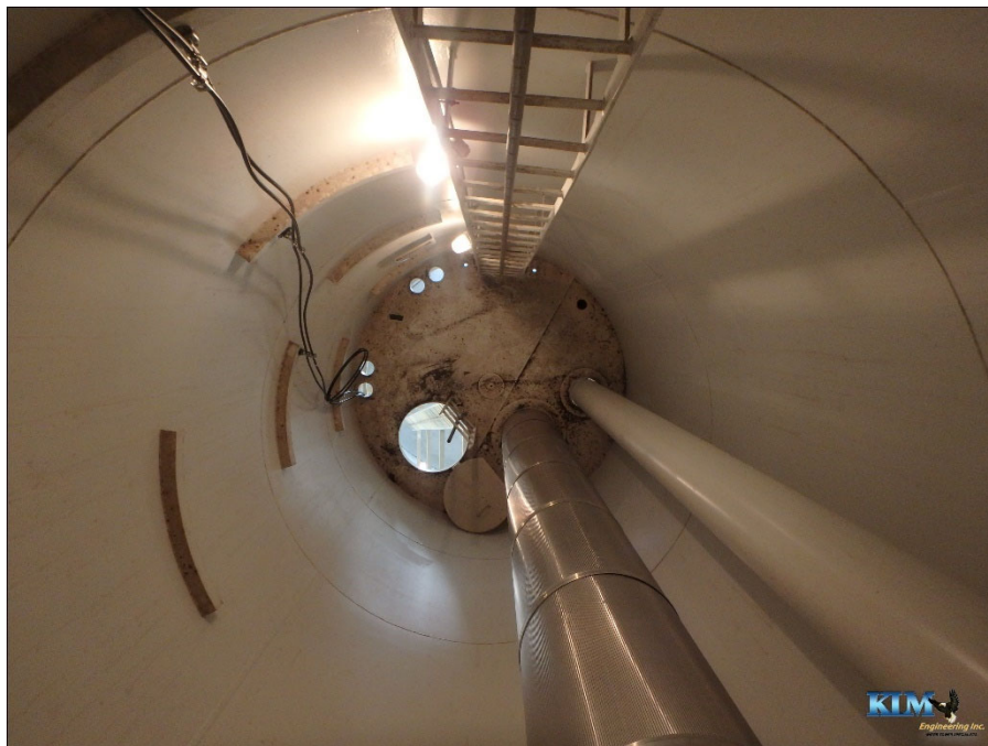
Photo No. 32 View of the pedestal and bottom landing
