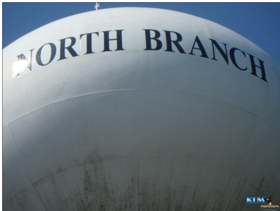
Photo No. 50 Water compartment and lettering
