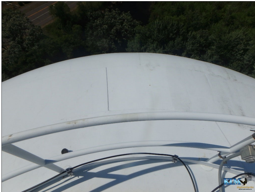
Photo No. 46 Condition of the roof and handrail
