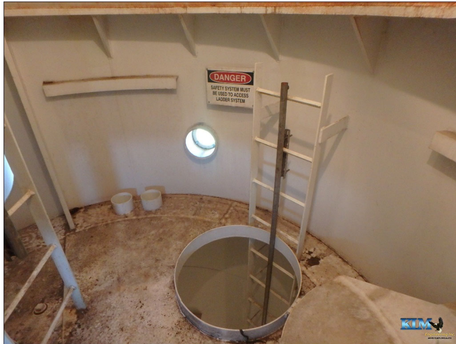
Photo No. 29 Condition of the top landing
