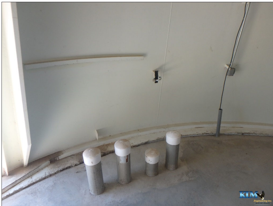
Photo No. 38 Condition of the base cone
