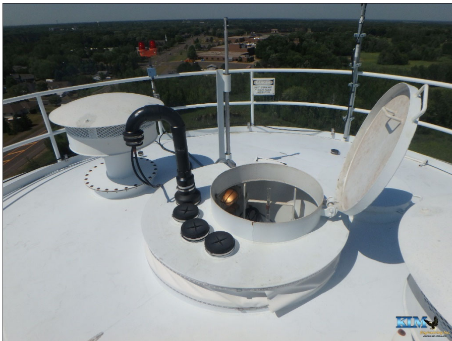
Photo No. 44 Top of the drywell tube, final vent, and handrail
