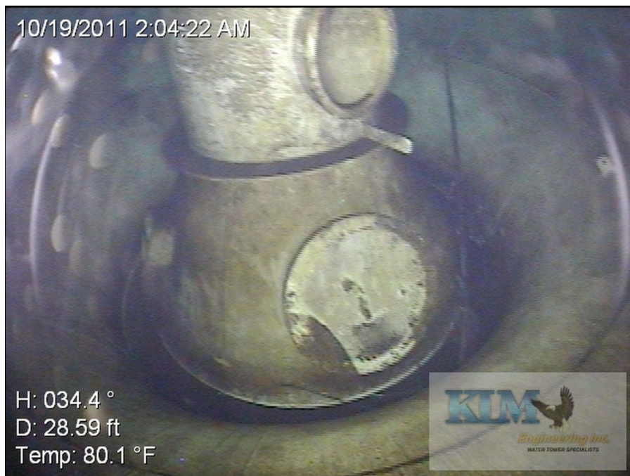
Photo No. 16 Access manways in the drywell tube and bowl
