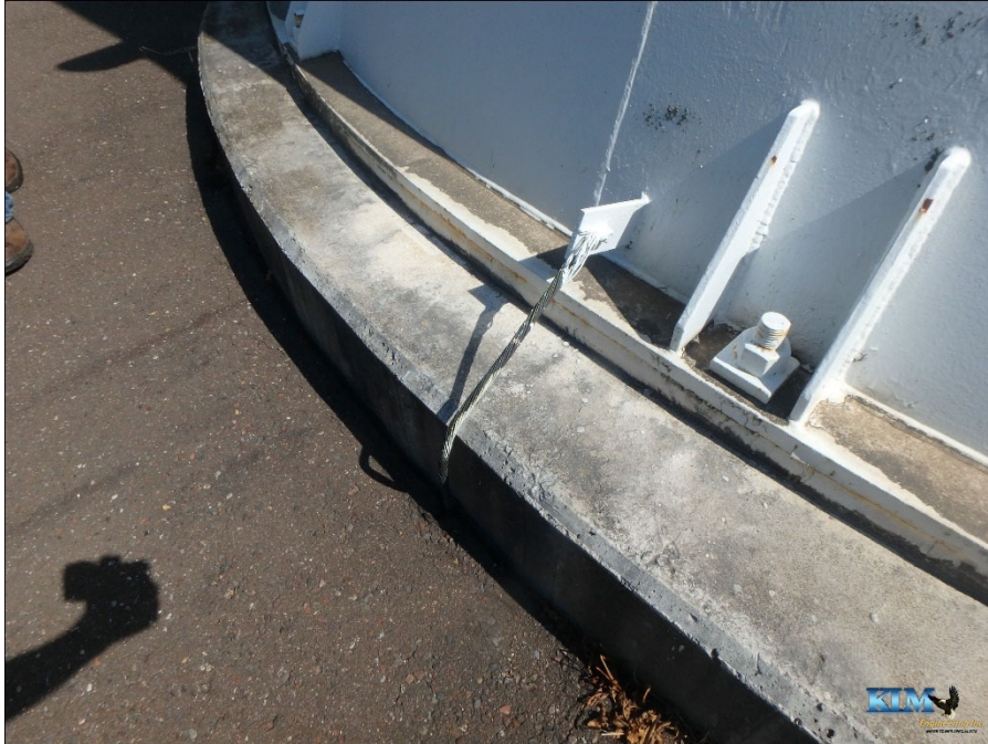
Photo No. 57 Tower base plate and foundation
