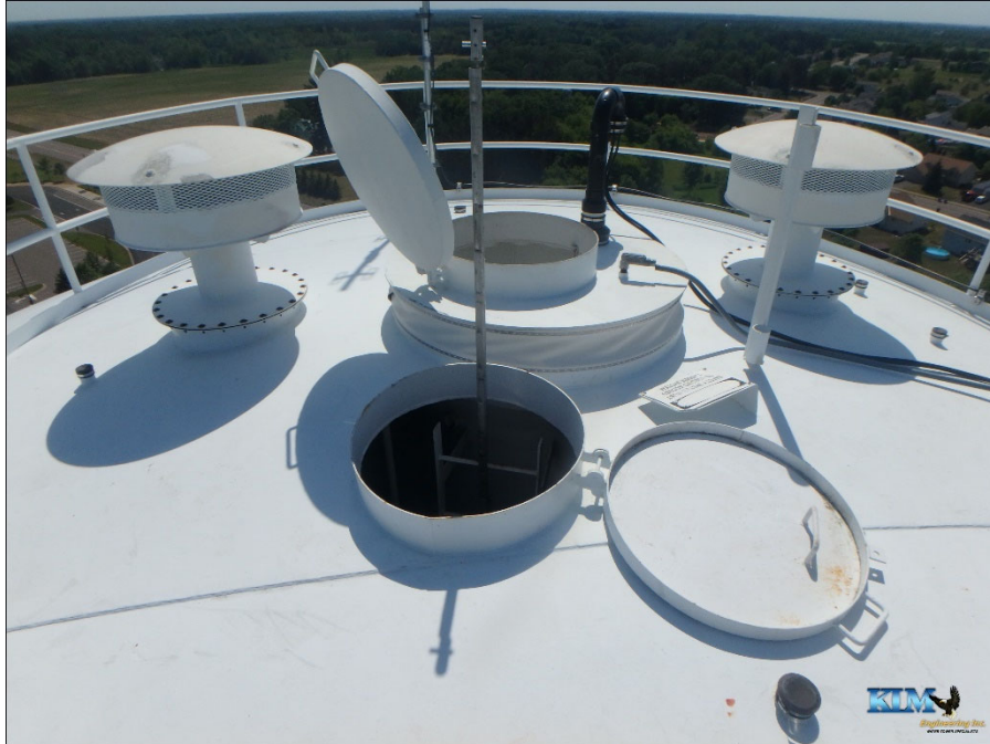
Photo No. 43 Overall view of the roof
