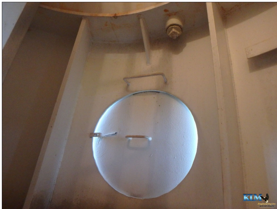
Photo No. 28 Painter's hatch
