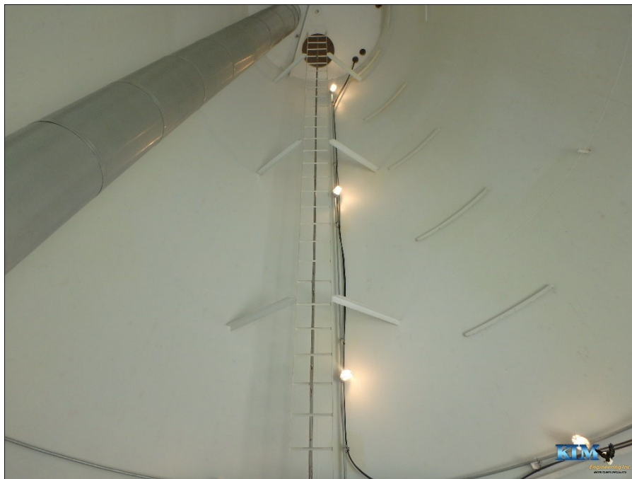
Photo No. 34 View of base cone and ladder
