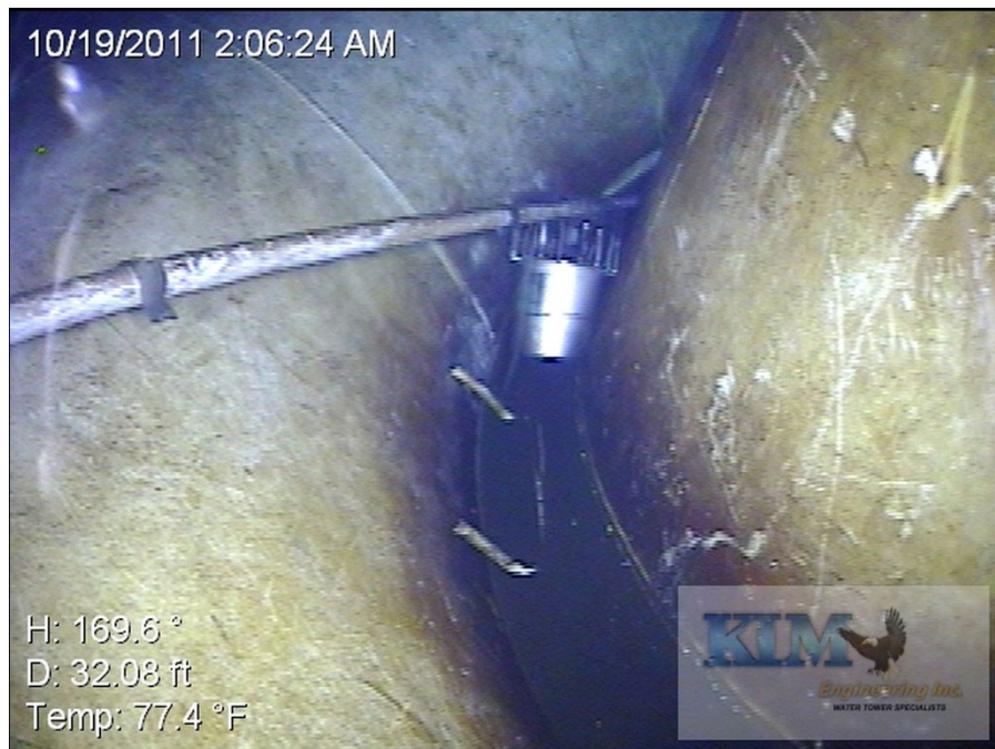
Photo No. 19 Fallen mixer and mount in bottom of the bowl
