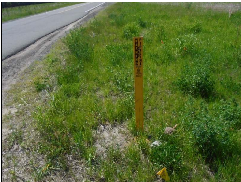
Photo 9: Looking west along 400 th Street from the southeast property corner at natural gas pipeline marker and gate valve cover.
