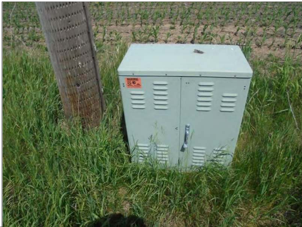
Photo 3: View of underground cable pedestal on the middle part of the west property line, looking east at Site.
